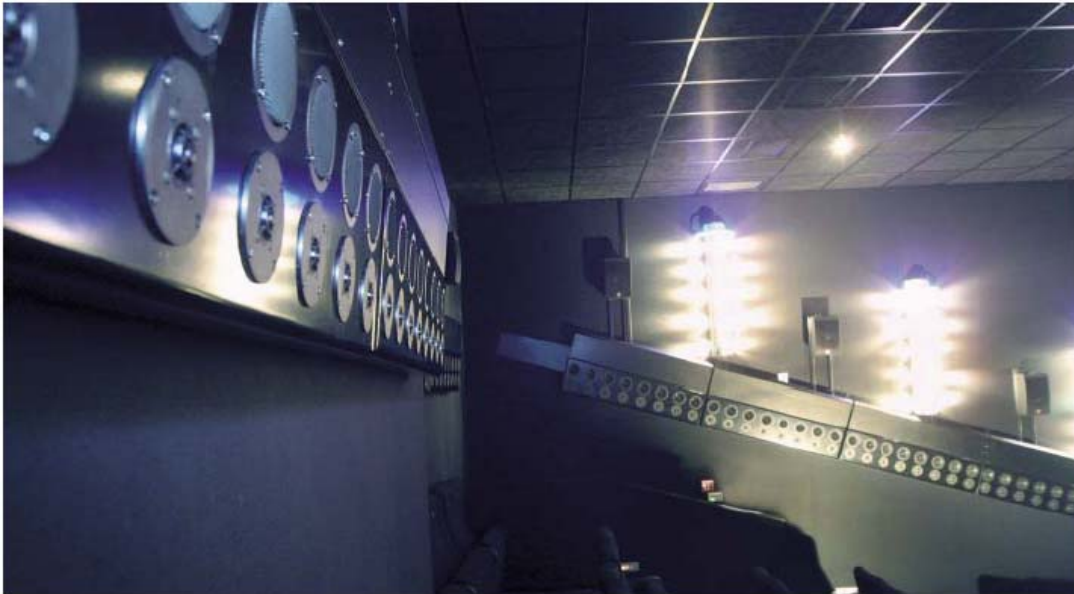
Figure 9-7: WFS speaker array in the Ilmenau Movie Theatre
